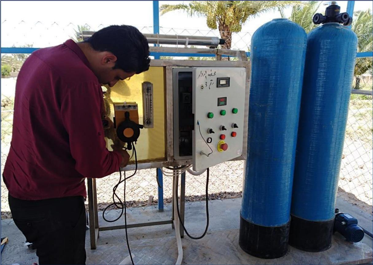
Installation of an RO Unit to purify the water provided by the newly constructed well in Al-Anbar
